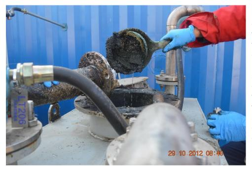
Figure 2 shows the collection of oil that is separated in the housing. In this case the oil is a heavy oil and the system was operated at 70° C to allow a lower viscosity oil to be separated. The concentration of oil can impair the solids separation however a method has been
